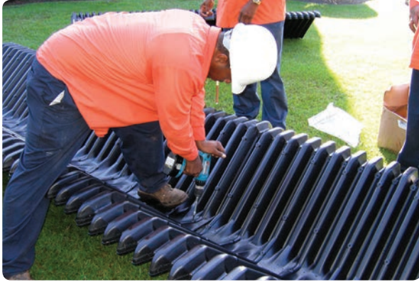
Self-tapping screws hold the channel together.
