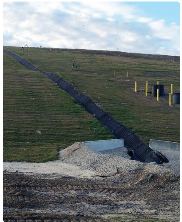
Vegetation grows up to the side of SmartDitch to minimize erosion.
