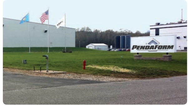
PendaForm is located in Portage, Wisconsin and operates 250,000 SF (23,230 SM), ISO certified facility.
