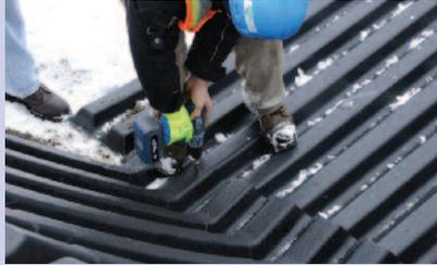
A handheld power drill is used to install the self-tapping, corrosion resistant screws that join each section.
