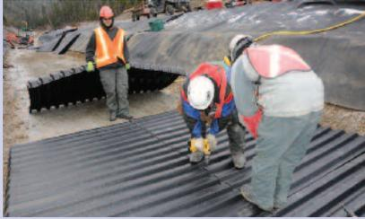
Weighing less than 75 lbs. each, the lightweight MegaDitch sections are easily moved into place.
