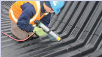
A water and weather resistant adhesive is applied to the seams between the base sections and the interlocking/overlapping sidewalls.
